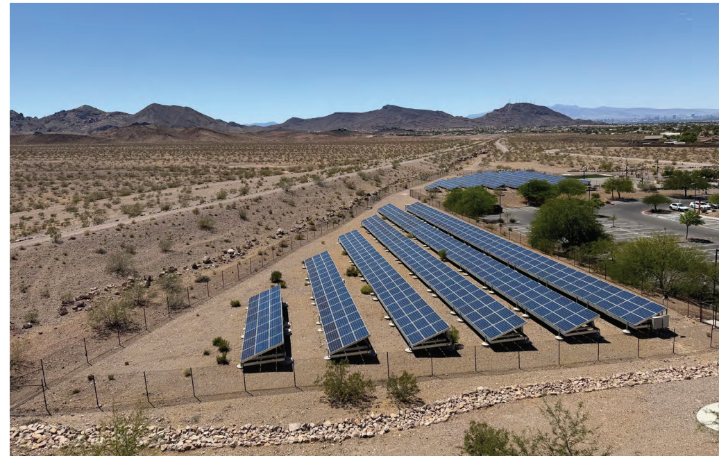
The University's existing solar array is a good visual representation of the institution's commitment to sustainability and energy resilience.
